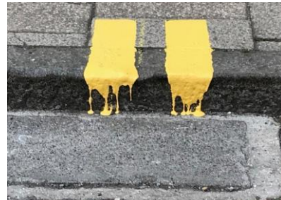
Road markings on the High Street
